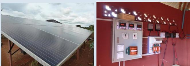
Thahara Pindaya is a new concept of small hotel permitted under new B&B laws that allow accommodation provision in properties of less than 10 rooms: the theme is a self-sustaining "eco" farmhouse. Owners have installed a solar PV system at a cost of approximately €13,000 supplied by a Yangon-based company. The system is running properly. In times of heavy clouds, a back-up petrol generator is used since the installed battery capacity is insufficient.
